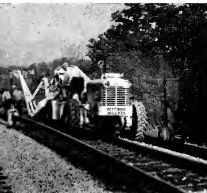
LAYING WELDED RAIL
